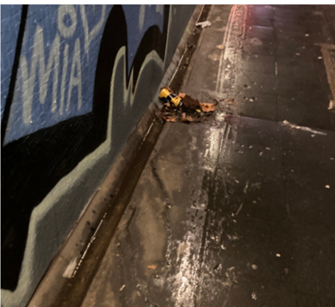
Drains are partially blocked by litter and leaves
