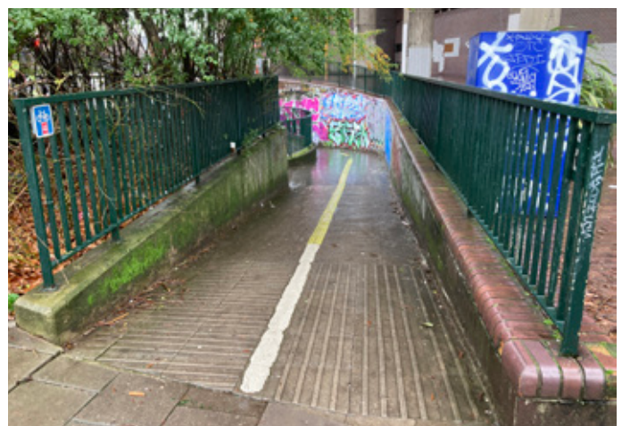
Very little signage at entrance to subway
