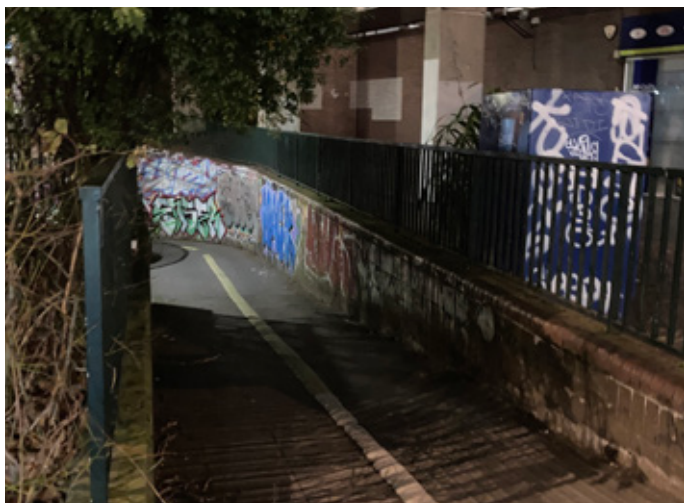
Lighting obscured by tree on the western approach
