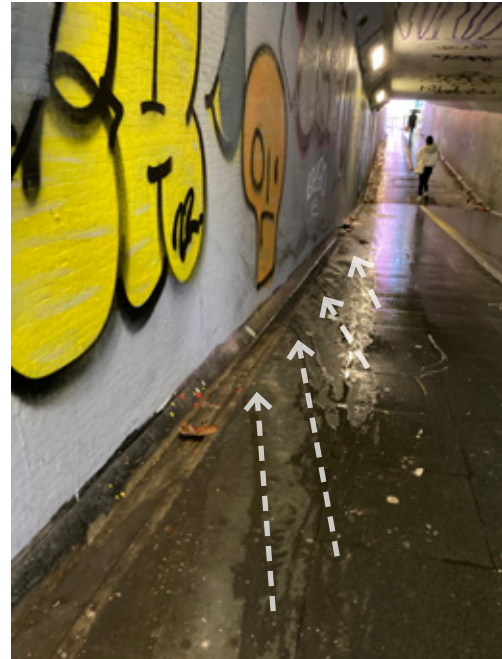
Rainwater run-off flows into subway and towards a drainage channel
